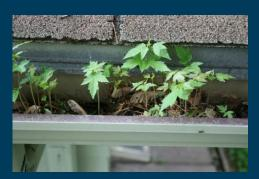
LEAVES, PINE NEEDLES, AND DEBRIS COLLECT AND CLOG OPEN GUTTERS
